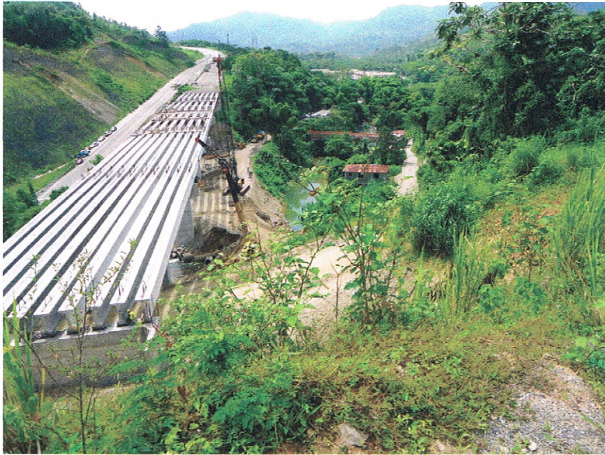
VIEW OF THE PROJECT END AND JUNCTION WITH AC-100065 (UNDER CONSTRUCTION)
